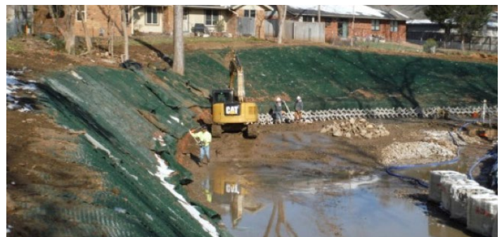
SOLUTION ARMORMAX® 75 was designed and installed for steep bank slope stability
