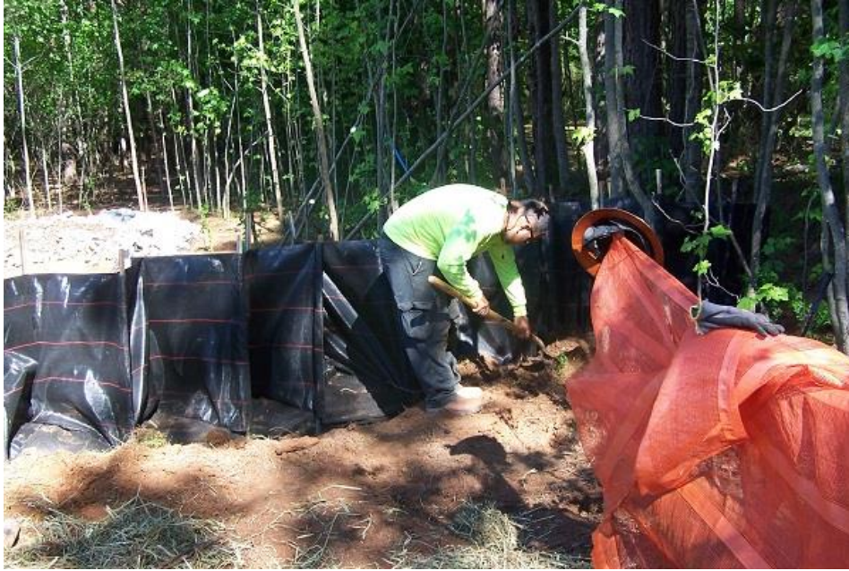
PHOTO 3 : CRAFS® installed across runoff flow path upstream of catch basin (5-2-17) ( Photo ID:100-0381LoPix )
