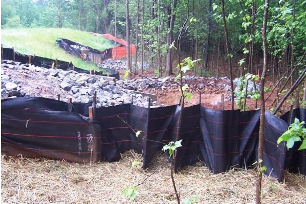
PHOTO 1 : CRAFS® upstream of catch basin after first rainfall event ... both installed the day before the rain ( Photo ID: 100_0401 LoPix )
