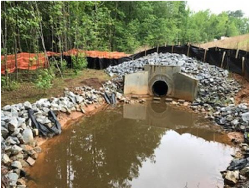
PHOTO 7 CRAFS® installed upstream of the retention pond to provide sediment retention and filtration before runoff enters the pond. Note the low turbidity level in pond maintained by CRAFS® upstream. (6-22-17) (IMG 0144 - LoPix)
