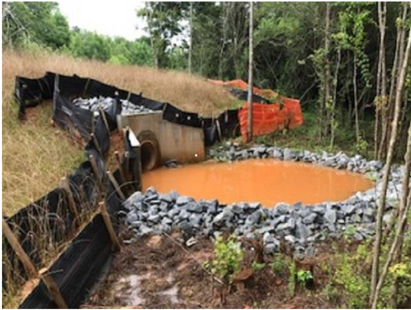
PHOTO 8 Second retention pond at same elevation and toe of same slope 150' away from CRAFS® protected pond (shown in PHOTO 7). (6-22-17) (IMG 0141 - LoPix)
